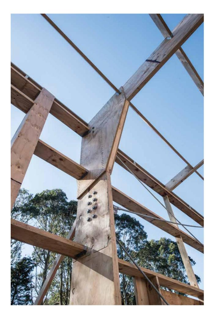
Using a hyFRAME® kitset also helped Max's contractors work smarter and faster. The offsite fabricated componentry and kitset construction process ensured accuracy of assembly, reduced build time and minimised the risk of construction errors compared to onsite fabrication of componentry.
