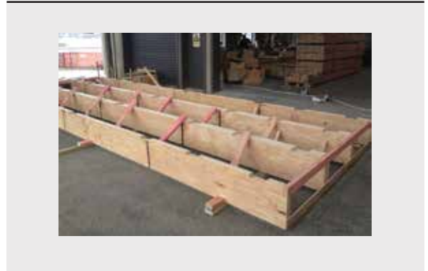
Photo 2: Fabricated Section (ex. Plywood Formface)
