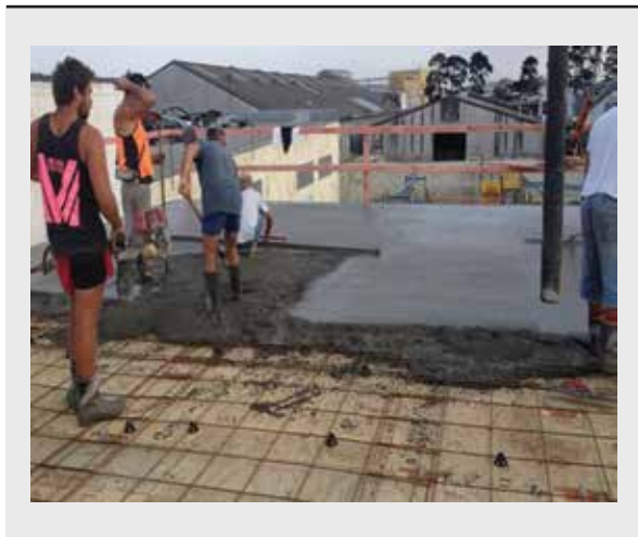
Photo 6: TCC Floor Laying Concrete Slab
