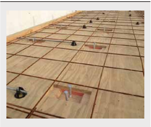
Photo 5: TCC Floor with Mesh Installed
