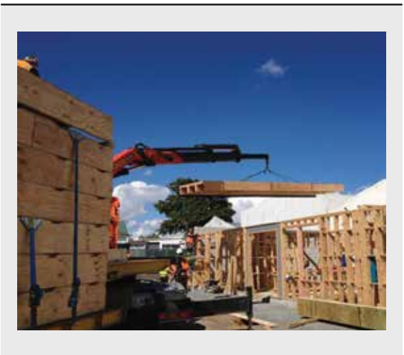
Photo 3: TCC Floor Delivery & Installation
