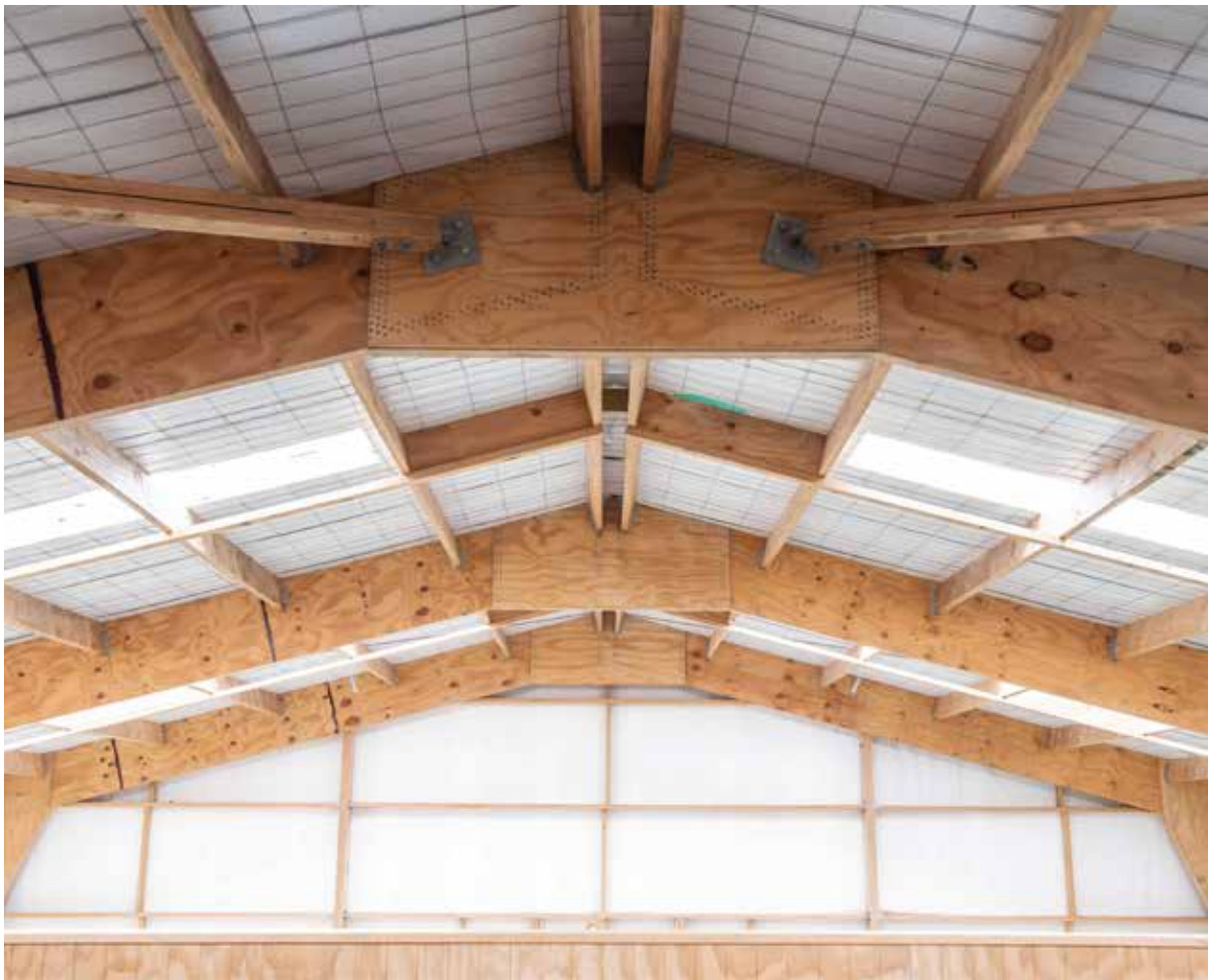
Manufactured from sustainably grown NZ plantation pine, rotary peeled, dried, and laminated together in continuous long lengths.
